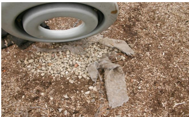
Tire Swing- Gravel exposed- Class B Hazard
