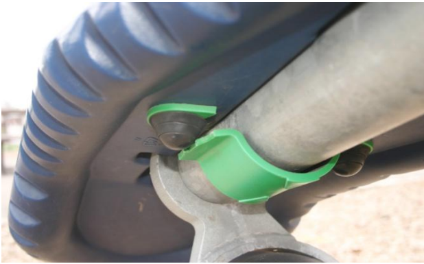
Climbing Structure- Rocking Tube- Gouges on Tires- MAINTENANCE
