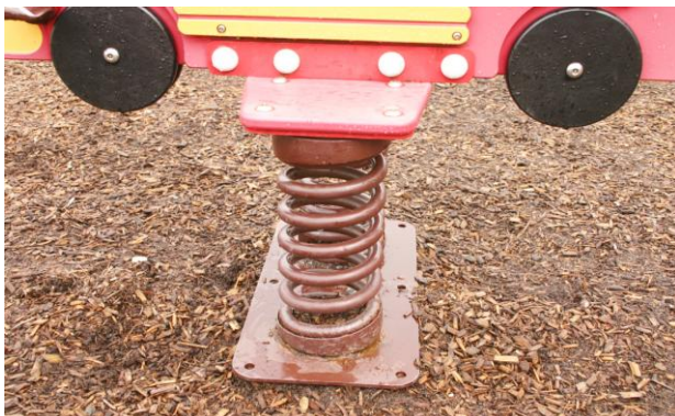
Fire Truck Spring Rocker- Loose at metal base plate- MAINTENANCE
