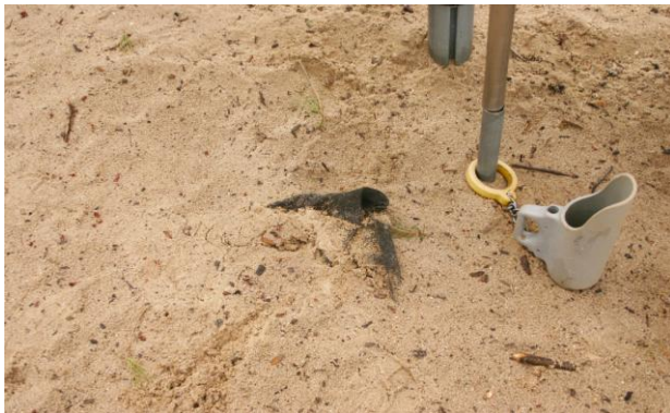
Fire Truck Spring Rocker- Loose at metal base plate- MAINTENANCE
