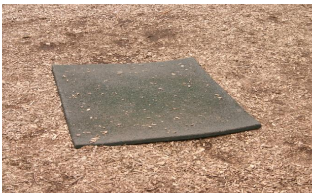
Tire Swing Set- Wear Mat Exposed- Class B HAZARD
