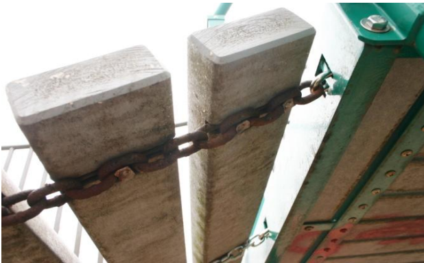
Metal Composite Structure- Chain Funnel Bridge- 4 Head Entrapments- Class A Hazard
