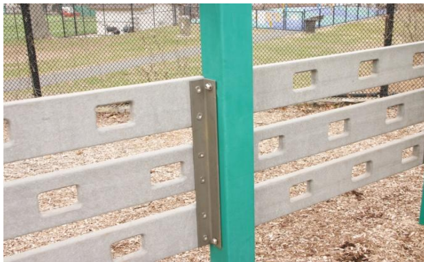
Metal Composite Structure- Suspension Bridge- 2 Head Entrapments- Class A Hazard
