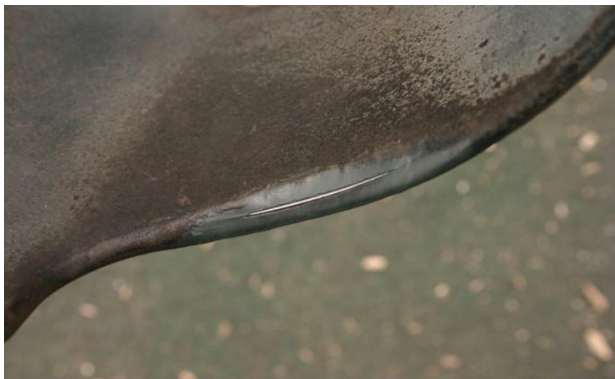
2 Bay Belt Seat Swing Set- Wear Mat Exposed- Class B HAZARD
