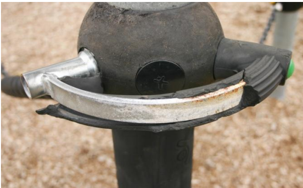
Climbing Structure- Climbing Steps Rubber Worn- MAINTENANCE
