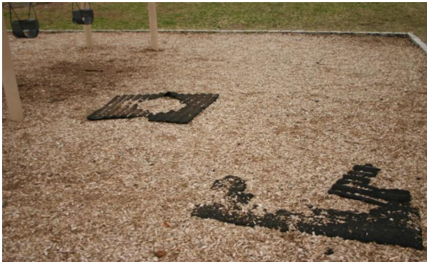
8ft Swing Set- Mats Exposed and damaged - Class B Hazard
