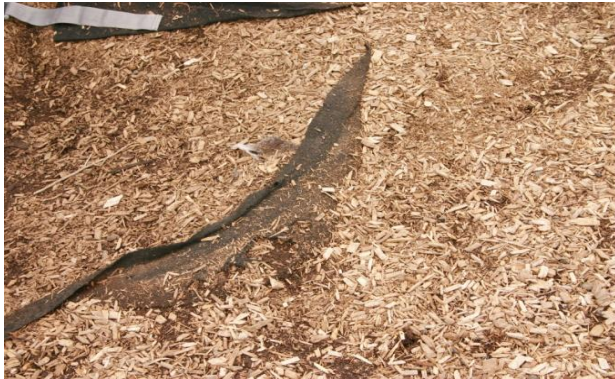
Antares Galaxy Climber- Holes in Rubber on Comets- Class B Hazard
