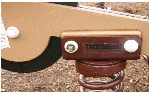
Motorcycle Spring Rocker- Bolt Cap Missing- MAINTENANCE
