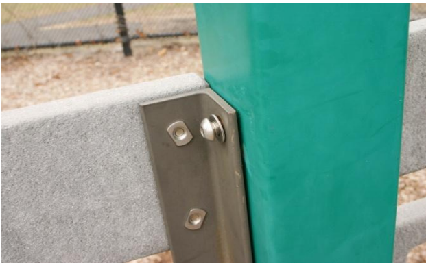
Metal Composite Structure- Climbing Wall- 2 protruding bolts- Class A Hazard
