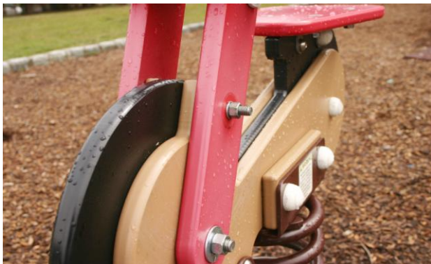
Motorcycle Spring Rocker- Bolt Cap Missing- MAINTENANCE
