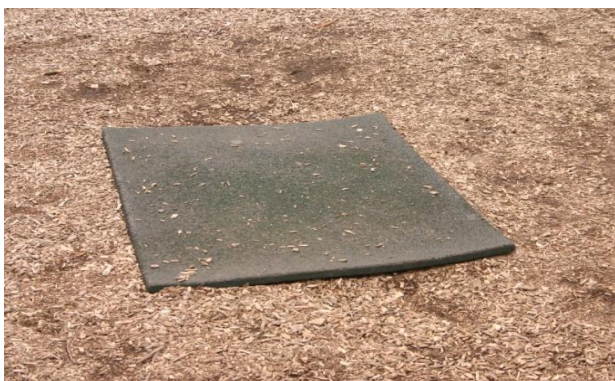
Tire Swing Set- Wear Mat Exposed- Class B HAZARD
