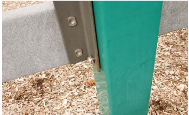
Metal Composite Structure- Climbing Wall- 2 protruding bolts- Class A Hazard
