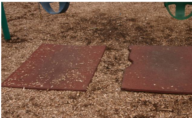
8ft Swing Set- Wear Mats damaged- MAINTENANCE
